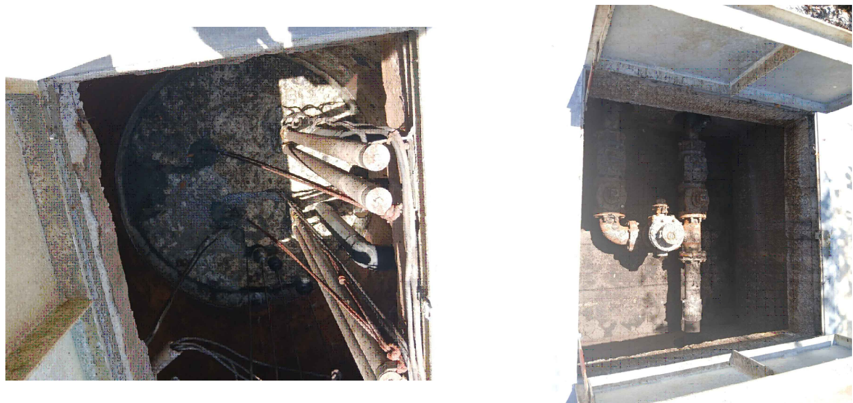
WESTERN WET WELL & VALVE VAULT
